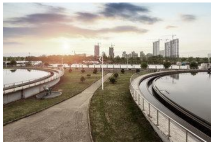
Waste Water Treatment
